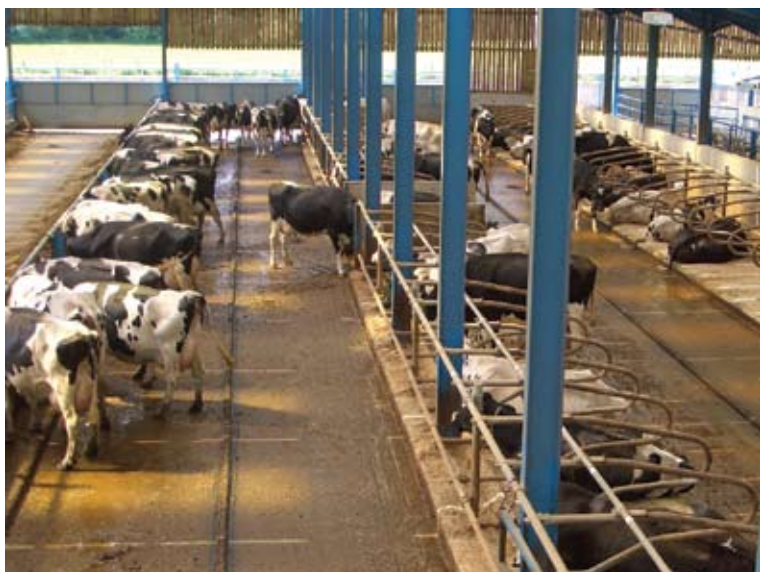
Cow housing at Wood Park Farm, University of Liverpool
